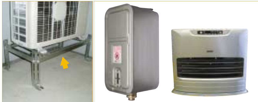
Trestle for outdoor unit of air conditioner (unpainted) Fuel tank for oil fan heater
