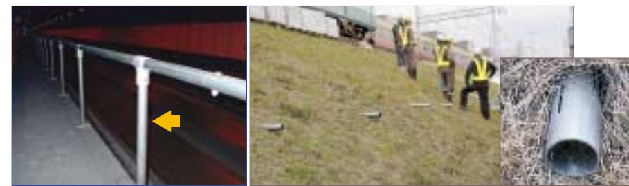
Handrail in tunnel
