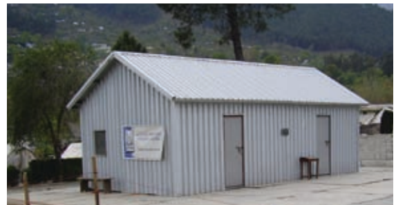
Using FRAMECAD technology, Metecno developed a simple 32 sq metre house that could be built quickly, economically and in large numbers to provide urgent relief following the 2005 Pakistan earthquake
